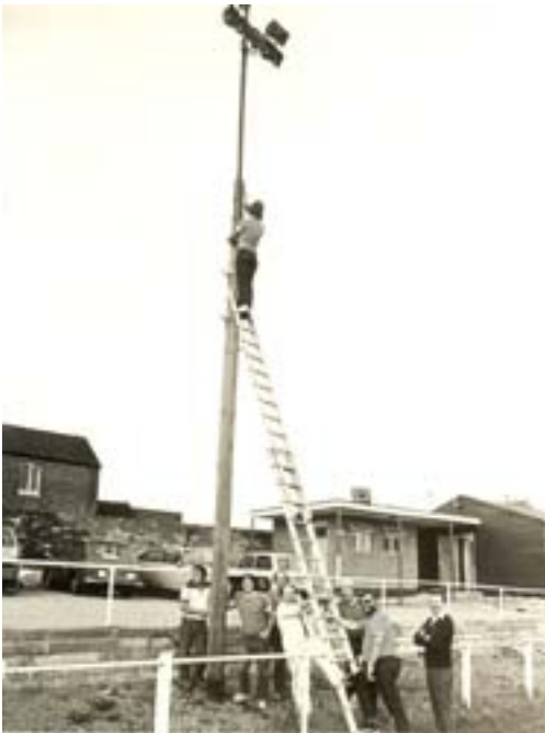
Installing the new floodlights
